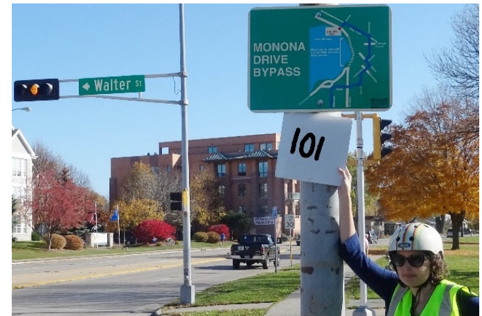
Figure 1-1: Including the sign ID number in a field work photo helps keep track of the signs in the inventory.
